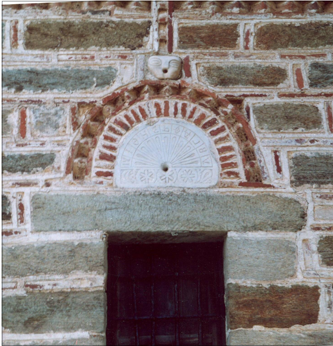
Fig. 2 The St. Lavrentios vertical sundial has been incorporated in the south wall of the main church (Catholikon) of the Monastery, symmetrically over the window's lintel.
