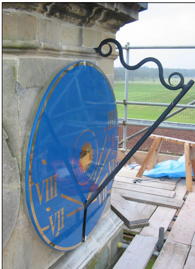
Fig. 7a. The north dial in position, but without the narrow gnomon access strip. Photo: M. Hollingsworth.
