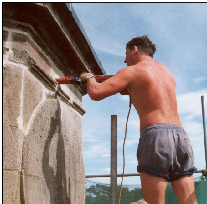
Fig 4. Drilling the large holes in the replacement stones for the “west” dial gnomon.
