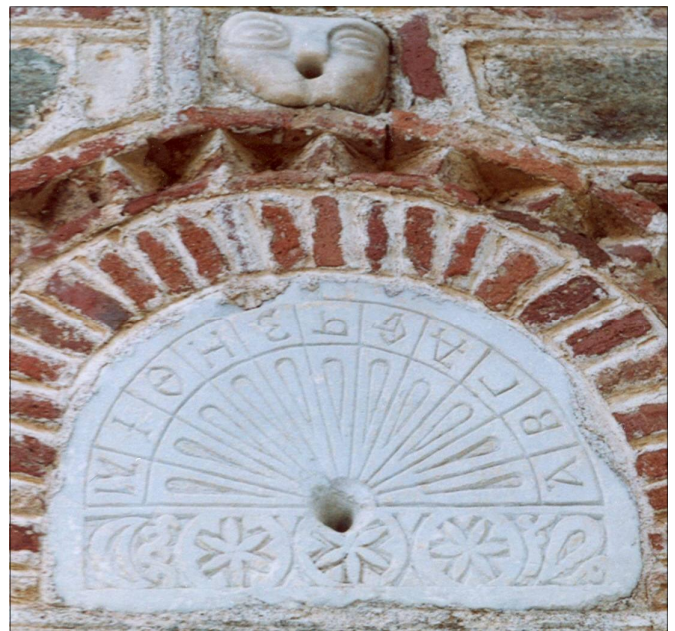
Fig. 3 A close-up of the sundial. Note the upside-down Greek numerals (letters), which contrast with the typical Byzantine decoration of red ceramics, and the ancient lion head above the dial plate.
