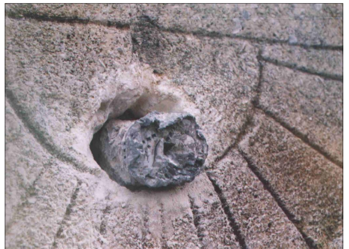
Fig. 3 Mortar-filled hole at the origin and loosened lead plug with rectangular hole at its centre.
