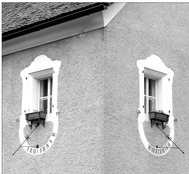
A pair of dials beneath windows in Weissbach, Austria.
